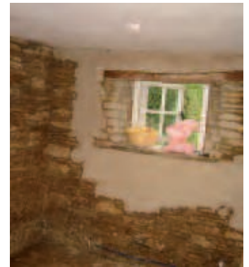
Exposing rubble walls to aid drying
