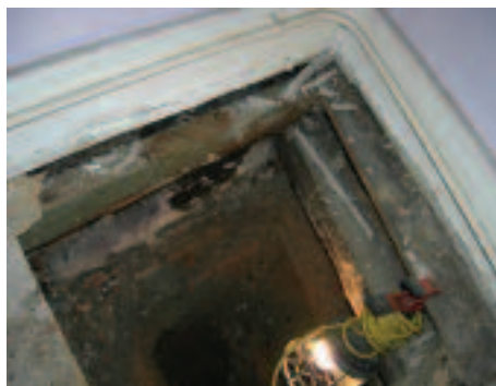
Sometimes internal trial holes are necessary to establish the cause of movement
