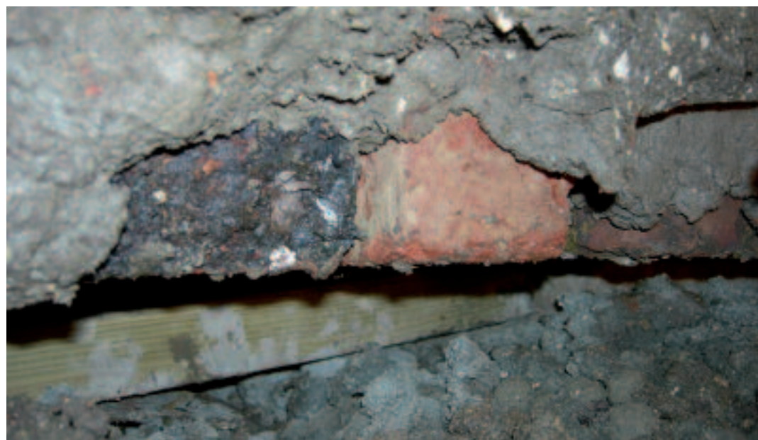
Timber packers in between original footing and concrete underpinning
